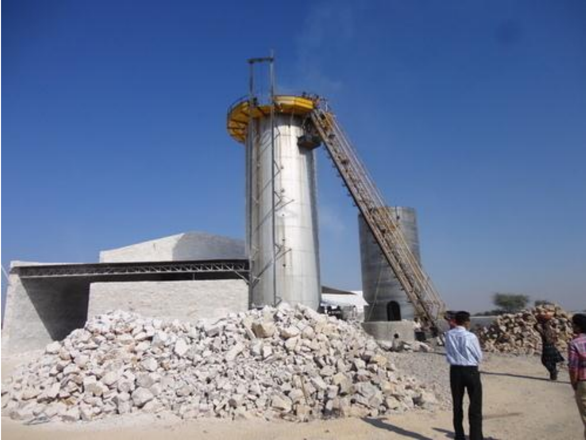
Lime vertical shaft kiln
