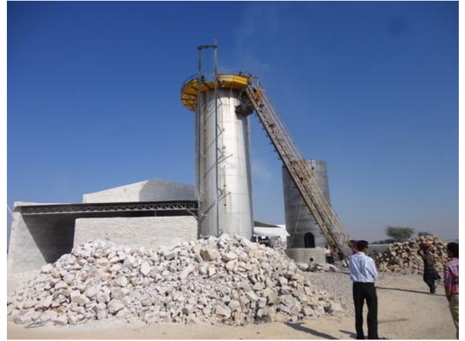
Lime vertical shaft kiln
