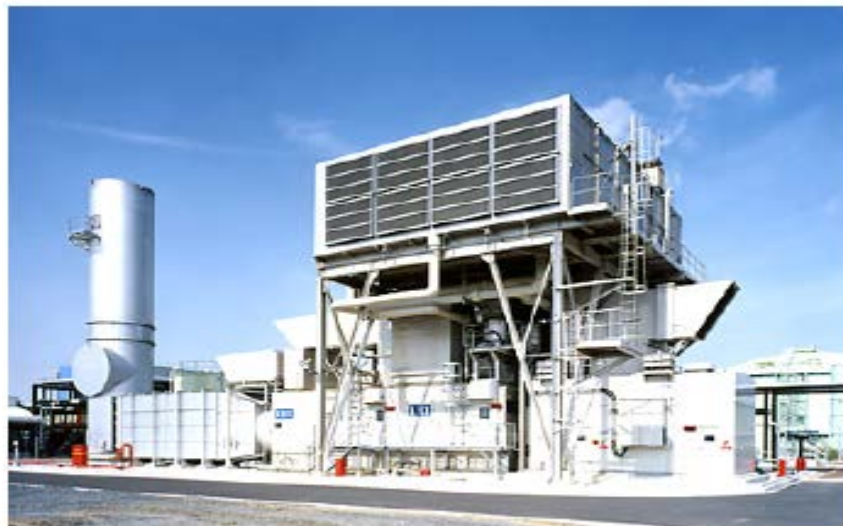
Figure 4. Typical simple cycle gas turbine power generator
