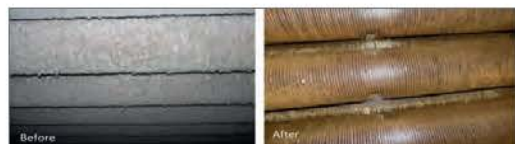
Figure 4 SMR furnace convection bank tubes before and after cleaning
