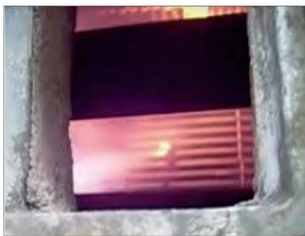
Figure 1a Small tube leak
