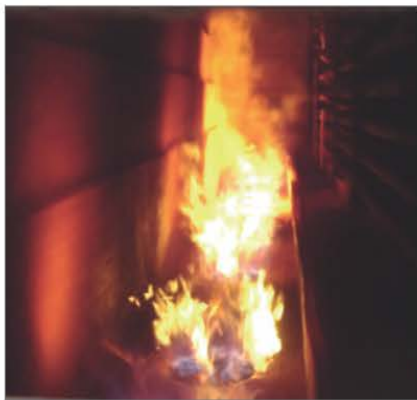
Figure 2a Refractory fallen onto burners
