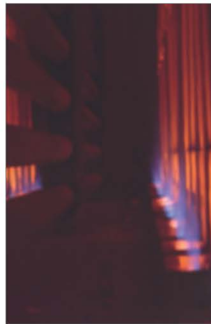
4b Clean firebox after adjustment
