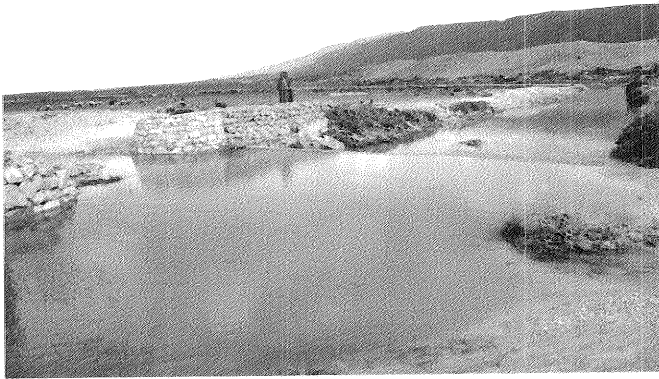
Water spreading structure in northern Tunisia provides supplemental irrigation water for wheat and other winter field crops.
