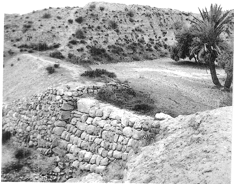
Jessour in southern Tunisia trap both runoff water and eroded soil but require maintenance to continue supporting high quality figs and olives.
