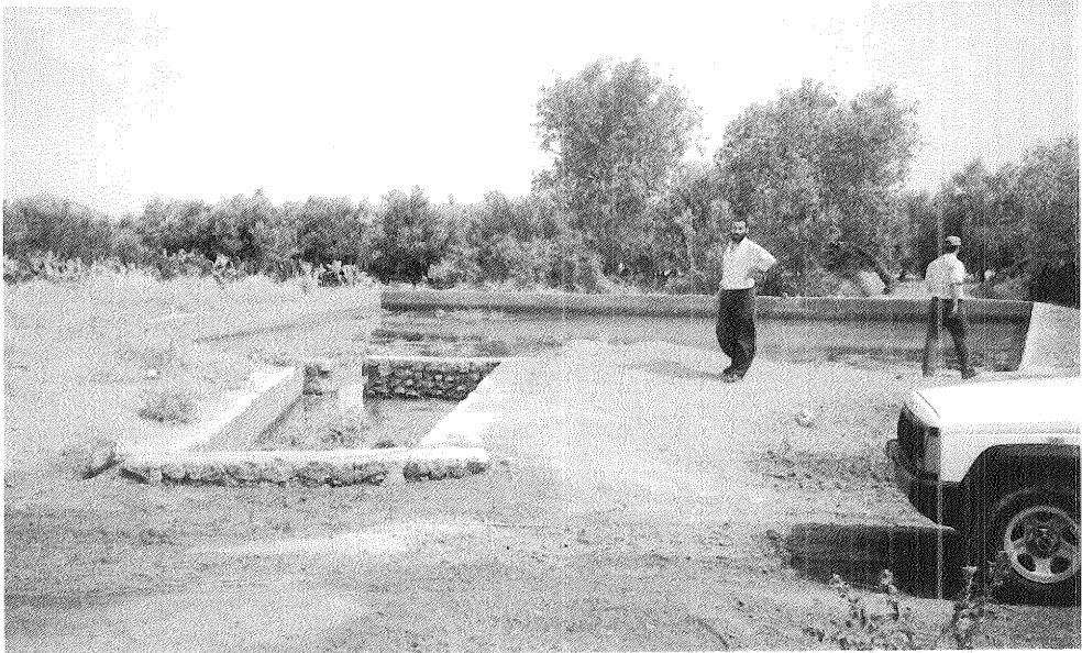
A low-flow-rate rhattara combined with a small storage basin for irrigation.
