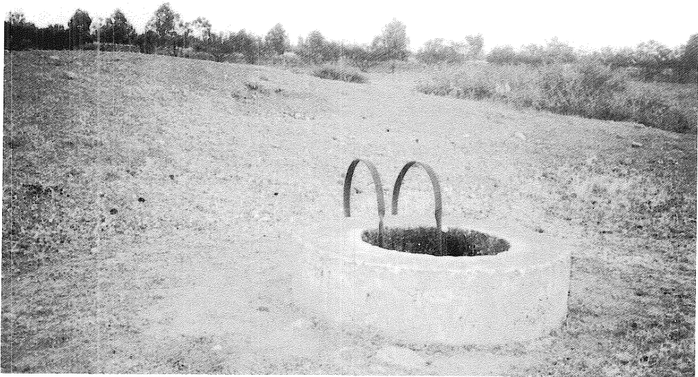
A vertical access shaft in a rhattara.
