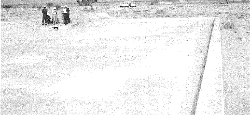
A fessoua providing drinking water to people and animals in central Tunisia.
