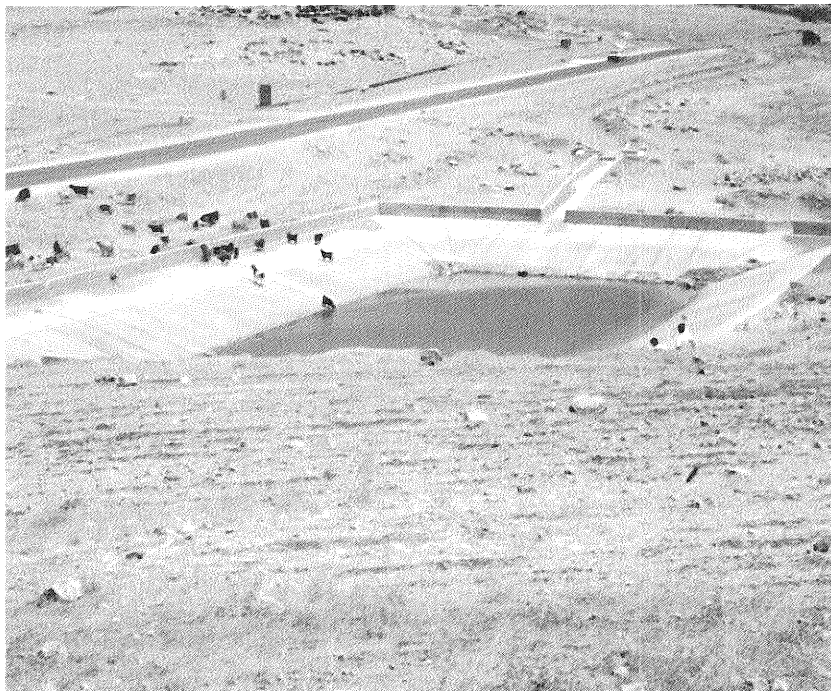
A water harvesting pond used by the Bedouins to water their animals in northern Jordan.
