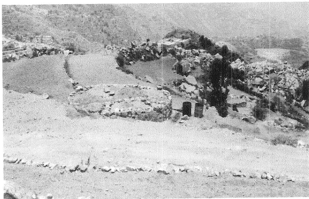
A siqaya under construction at Saper Mountain, Taiz.
