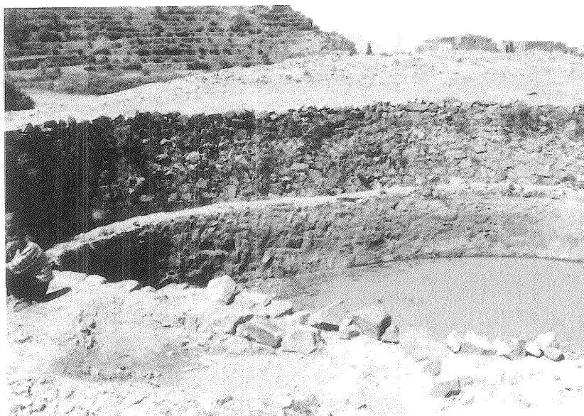
A karif providing water for livestock and for some household uses, at Saper Mountain, Taiz.
