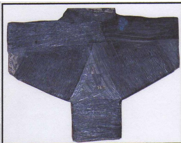
Fig. (13): Cracking pattern of corbel C5
