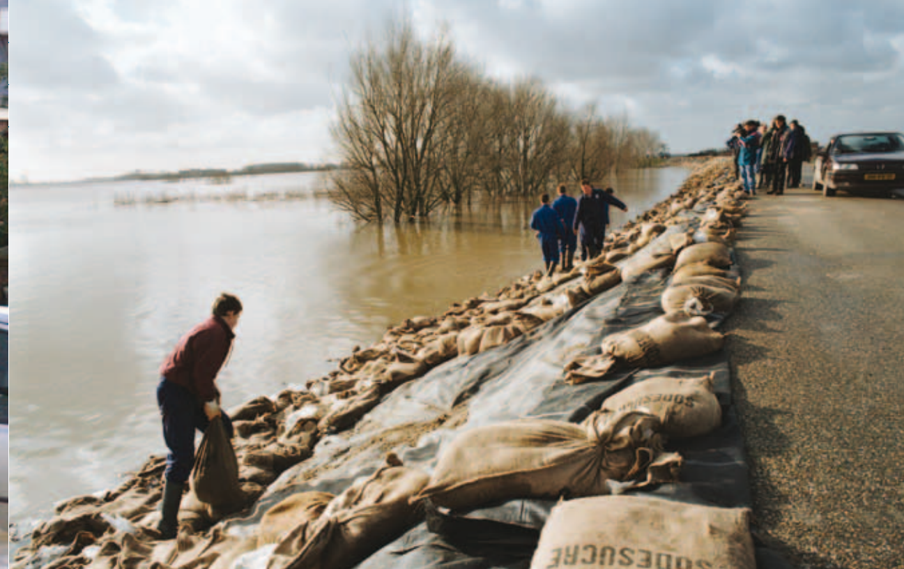
Emergency repair during high water at Ochten, The Netherlands in 1995
