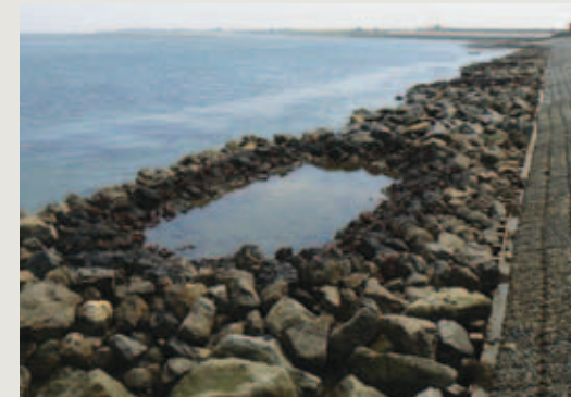
Ecobasin at the toe of a dike
