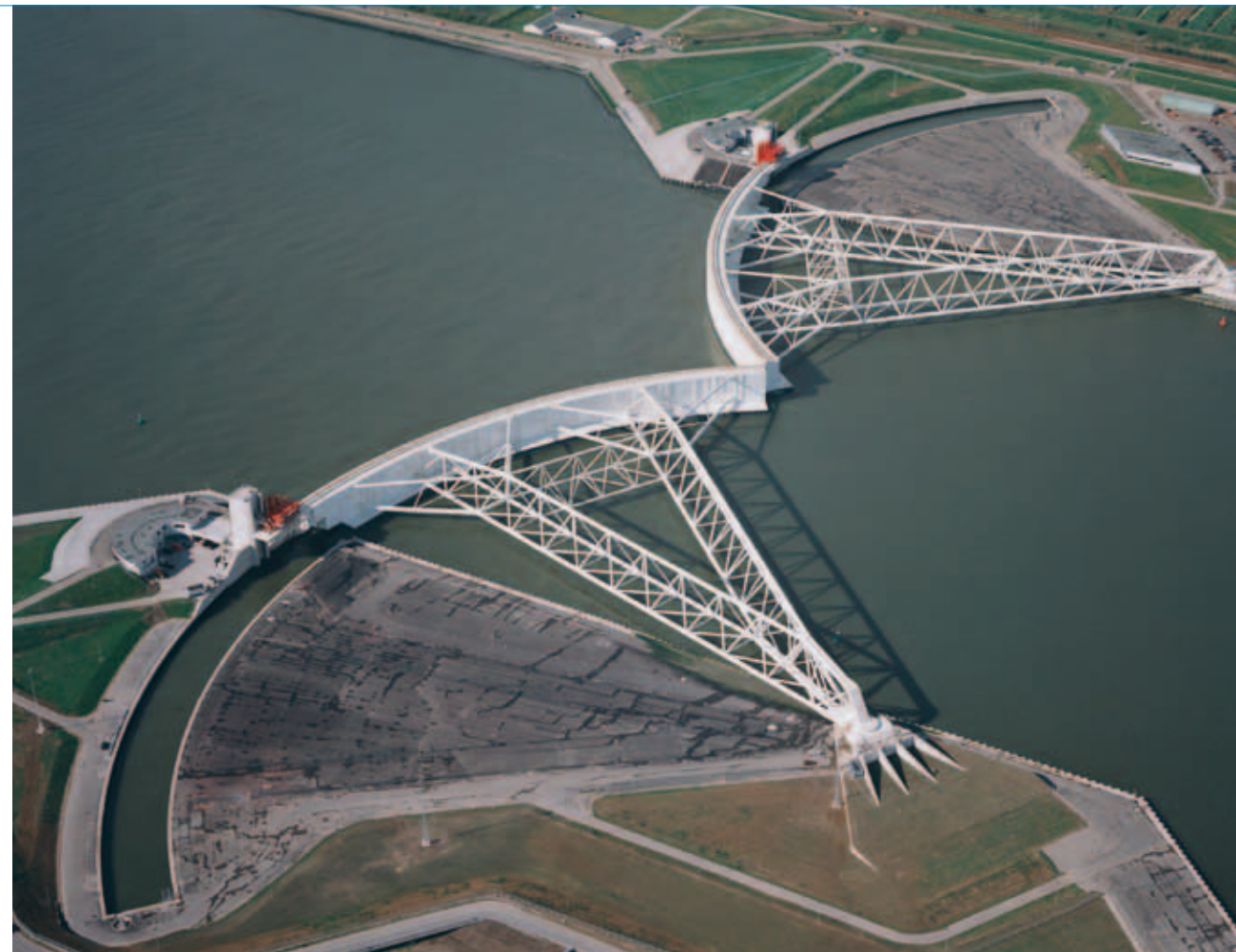
Maeslant storm surge barrier in closed position
