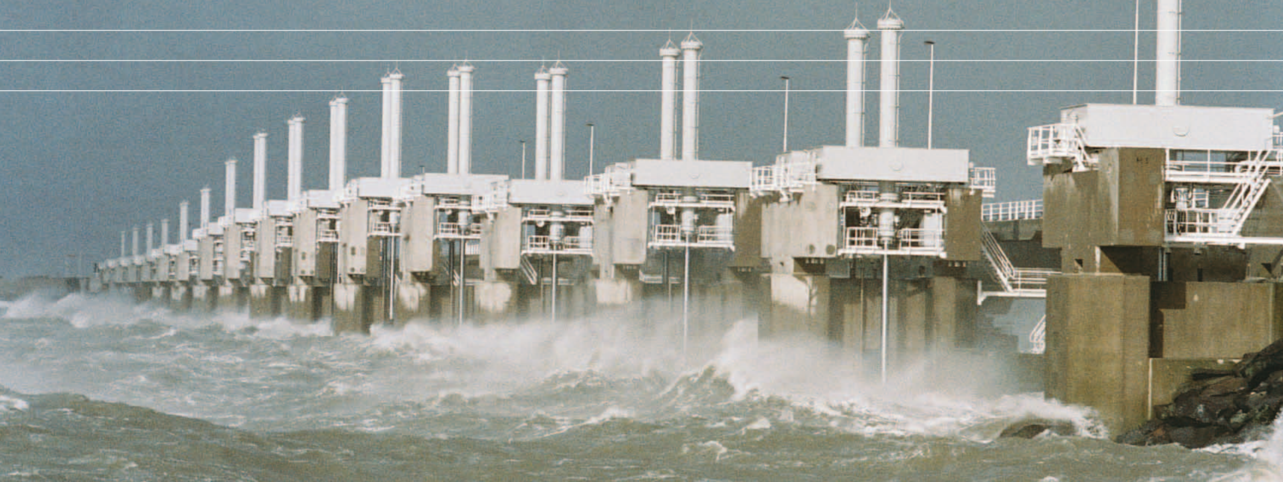
Oosterschelde storm surge barrier The Netherlands closed during heavy storm
