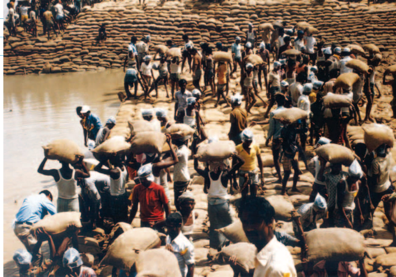
Repairing a dike breach in Bangladesh
