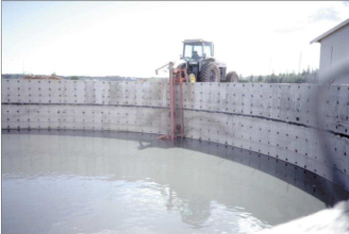
Liquid manure storage - circular concrete tank.
