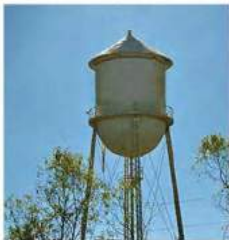
The center of gravity of this water tank can be determined by dividing it into composite parts and applying Eqs. 9-6.
