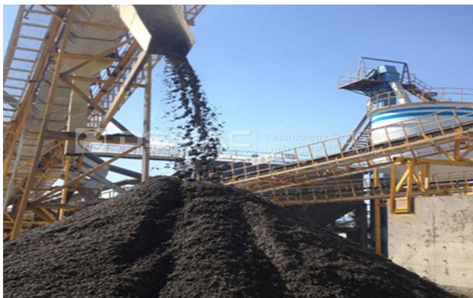
Coal line crushing
