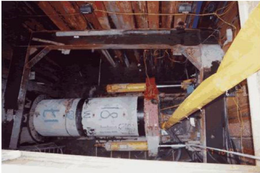
Hydraulic Jacks at Starting Pit
