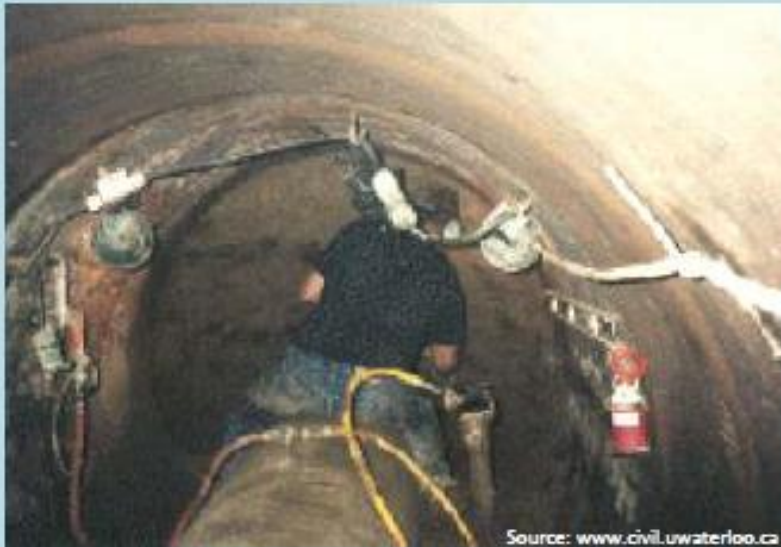
(a) Manual Excavation
