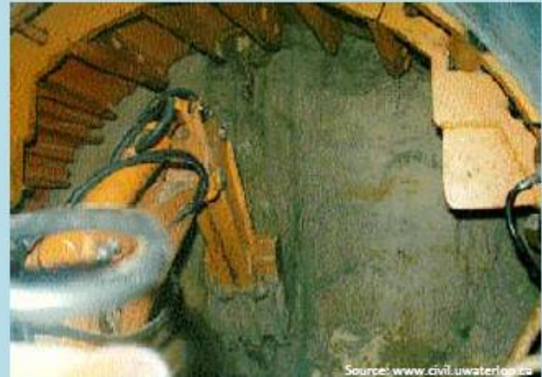
(b) Machine Excavation
