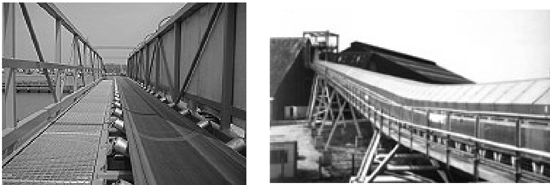
Fig. 6.1.11. Photographs of long centre conveyors with their structures
