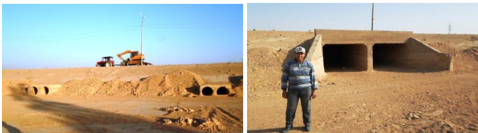
Fig (7): Field photographs showing the protection systems at Cairo – Aswan road (22/11/2018).
