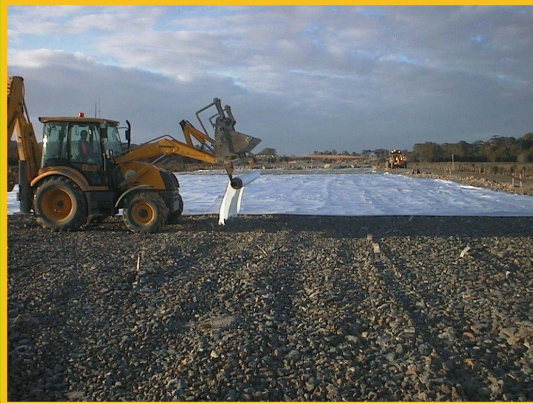
Geofabrics used on Pacific Highway
