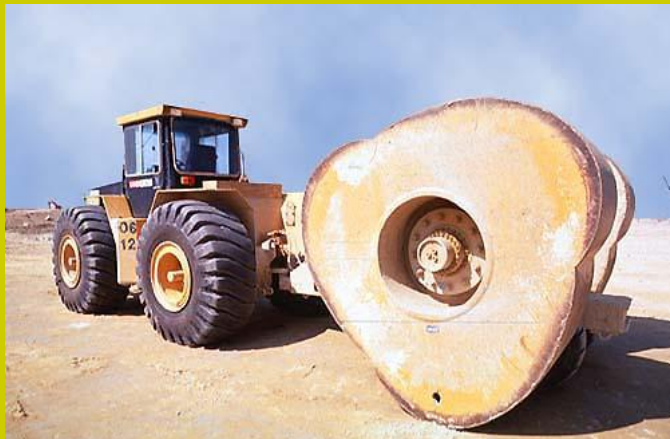
Impact Roller to Compact the Ground
