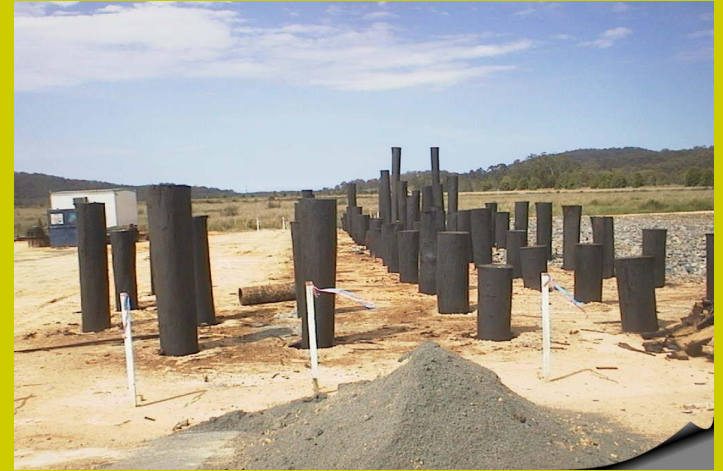
Driven timber piles, Pacific Highway
