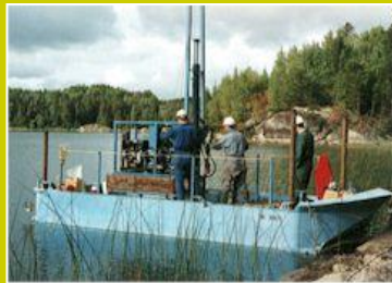
Water Boring from Barge for Bridge Crossing
