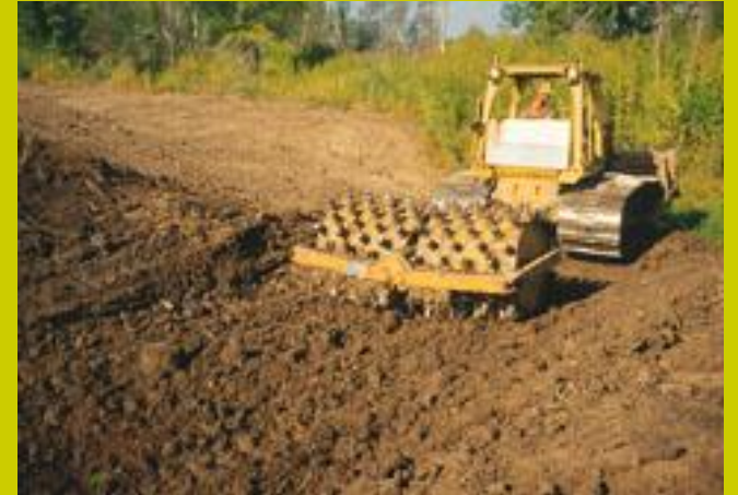
Sheep foot Roller to Compact Clay Soils
