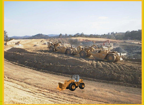
Roadwork, Pacific Highway
