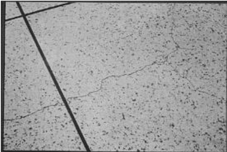
Floors tiles Workmanship-base concrete-grading of aggregate
