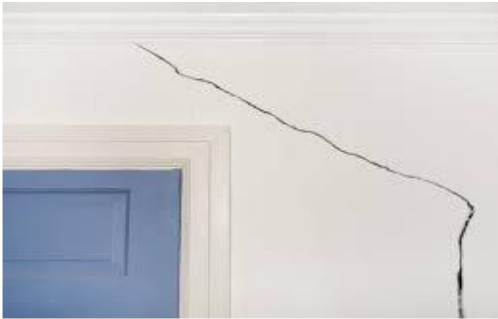
Internal wall - settlement of the floor
