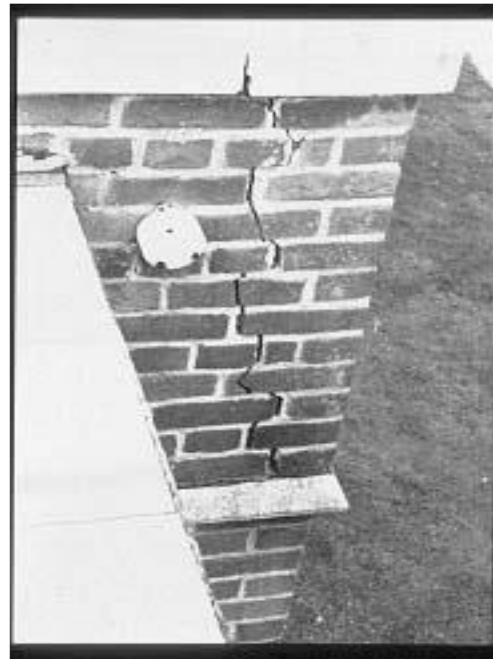
Wall cracks- Poor detailing-weak bond -diagonal stepped crack
