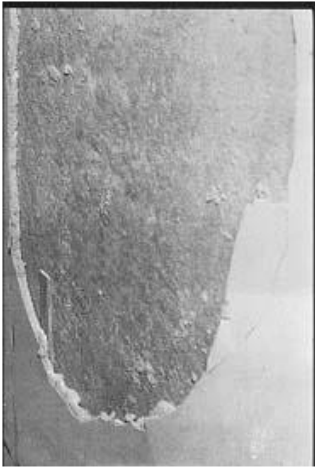
Plasterwork Workmanship-plasterwork on dense concrete
