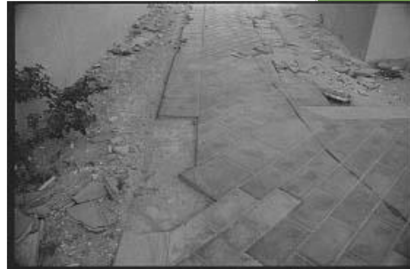
Floors tiles Workmanship-base concrete-grading of aggregate
