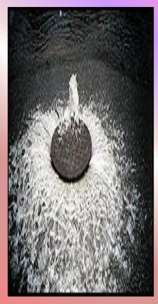
A manhole cover unable to contain a sanitary sewer overflow.
